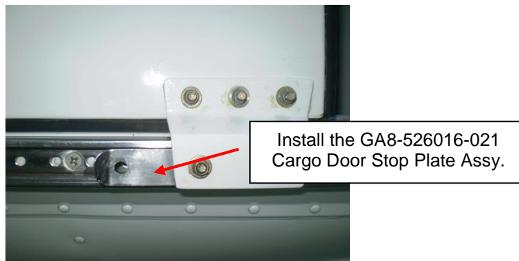
Figure 8: Fwd Door Stop Installation
